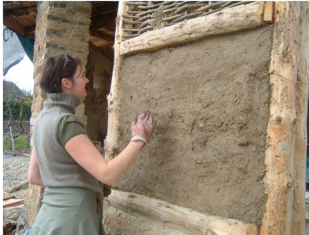
Figure 9. Wattle and daub earthen building (TC, 2007).
