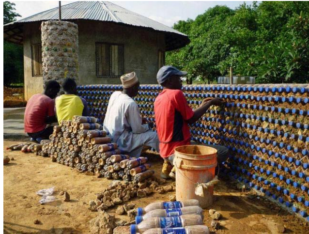
Figure 12. Plastic bottle construction (Hattam, 2011).
