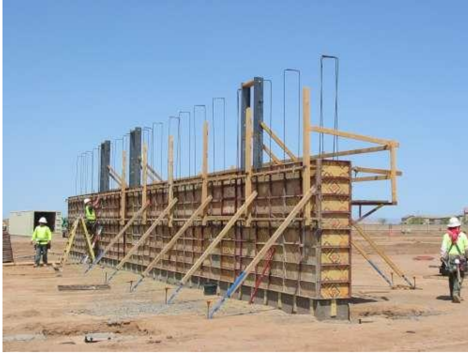
Figure 11. Rammed earth formwork (CAC, 2014).
