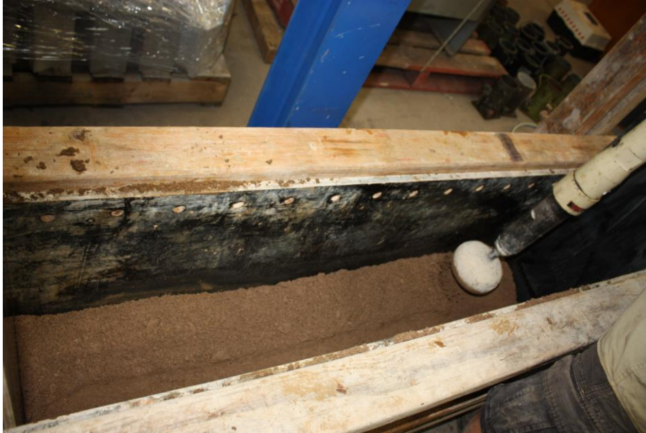
Figure 32. Compacting layers of soil between formwork (Netherton, 2015).
