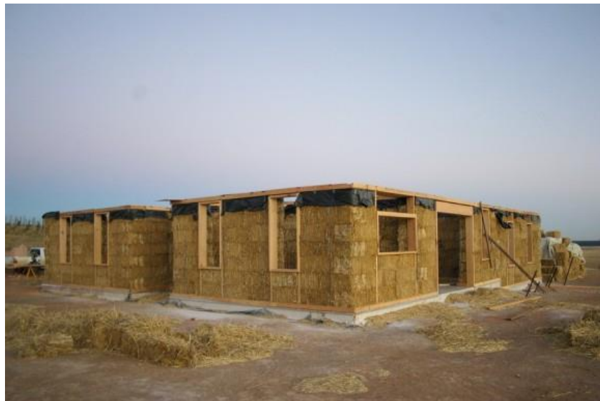
Figure 5. Straw bale construction (Glassford, 2015)
