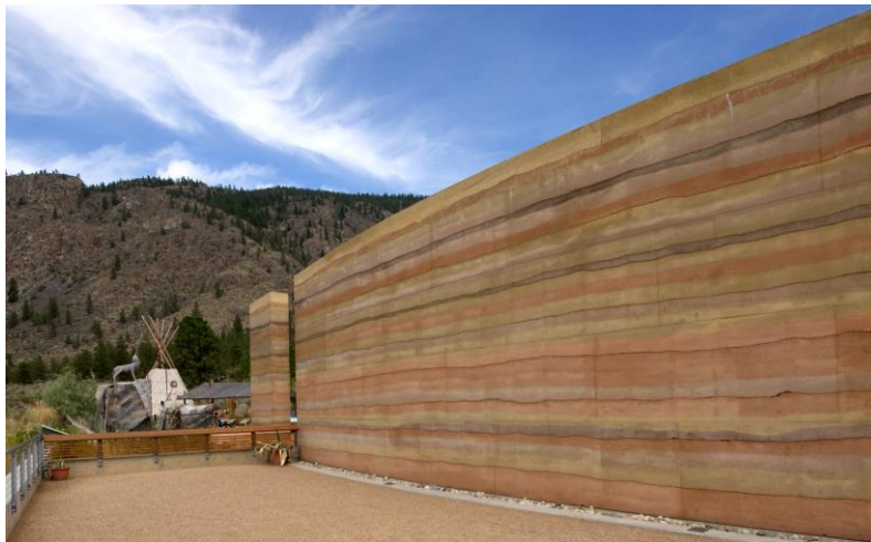
Figure 10. Rammed earth wall (RESHI, 2015).
